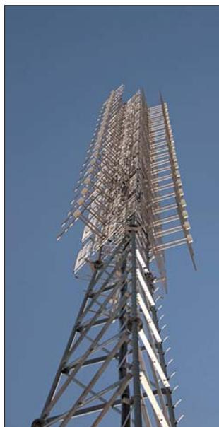
The Shively Panel antenna mounted on the tower.
