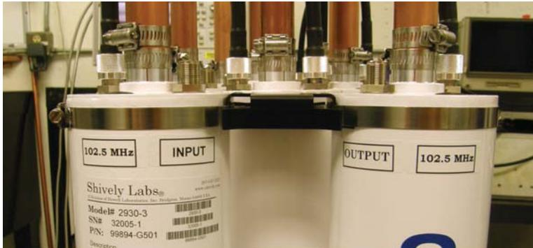
Figure 1. Identification of the ports and transmitter frequencies.
